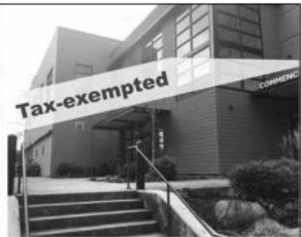
Location: 600 Franklin Street, Olympia Walker John
