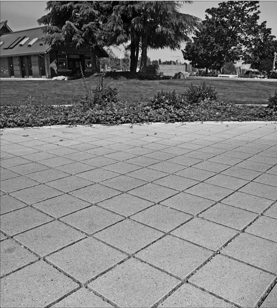
Permeable paving surfaces have been demonstrated as effective in managing runoff from paved surfaces. The photo above is of a parking lot at Percival Landing made with pervious pavers that allow rain to pass through the pavement into the ground. Photo: Robert Whitlock
